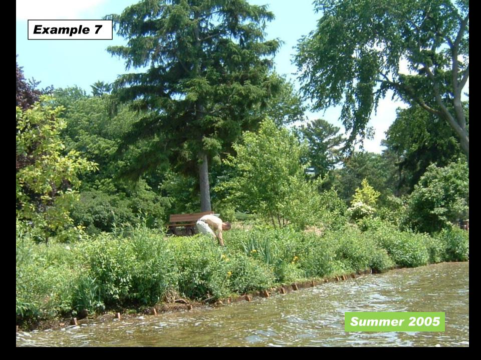
Problem: Eroding bank after removal of trees along shoreline. Solution: Bioengineered live crib wall w/ shrubs.
